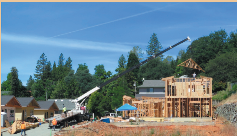
Roof trusses being lowered into place on Shadow Wood new houses in early June. Photo by Alan Shuttleworth
