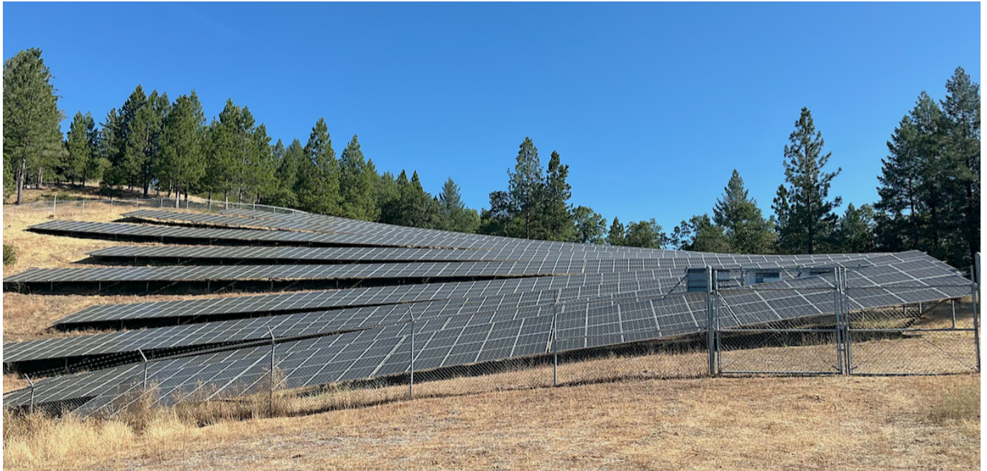
Waste Water Treatment Plant solar power array project completed.
