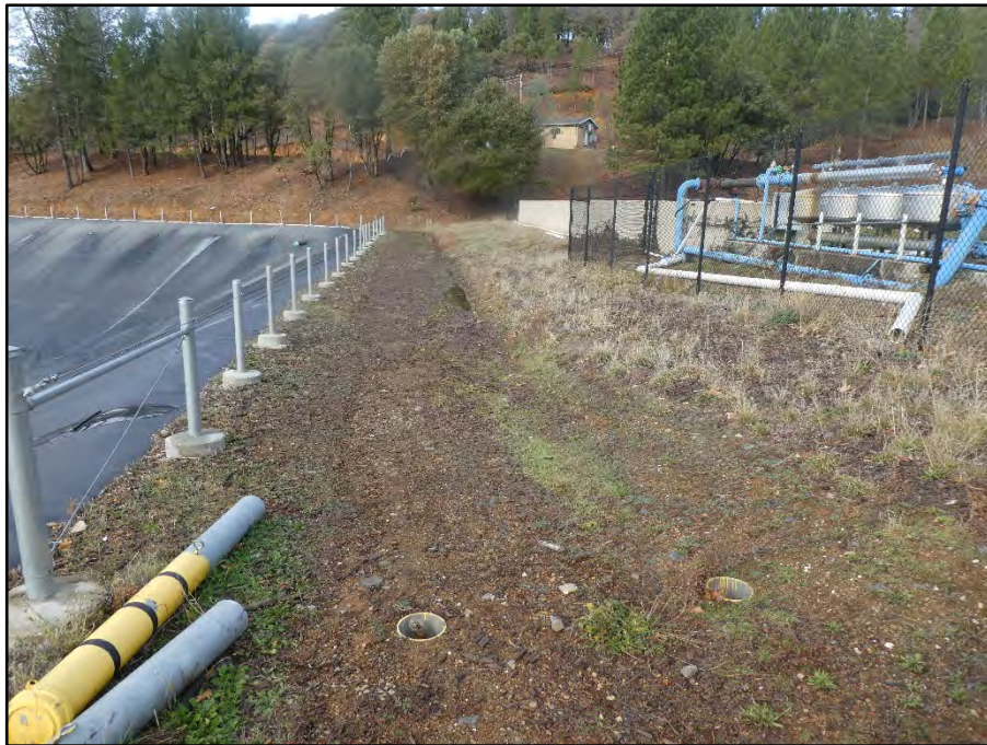
Looking west across area between Ponds 2 and 3 toward DAF/SAF System. Photo Date 01-15-20.
