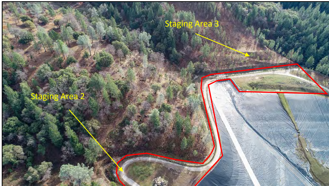
Looking south over proposed Alternative 2 and Alternative 3 sites in the southern portion of the WWTP study area. Photo Date 01-15-20.
