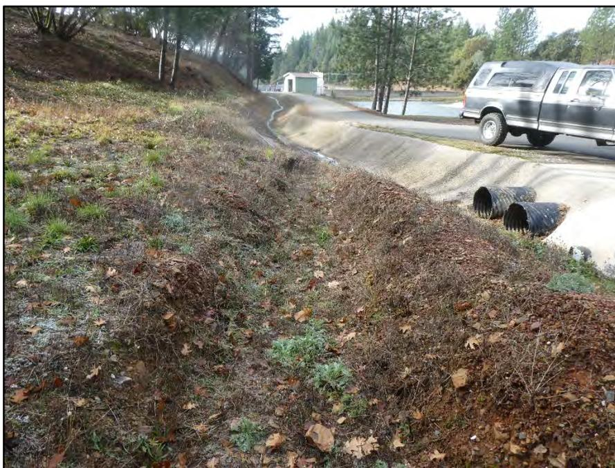
The ephemeral stream drains into a concrete lined channel along the eastern boundary of the WWTP area.
