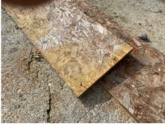
FIGURE 11 – DETAILS – 3” NAILS STICKING UP ENDANGERING KIDS
