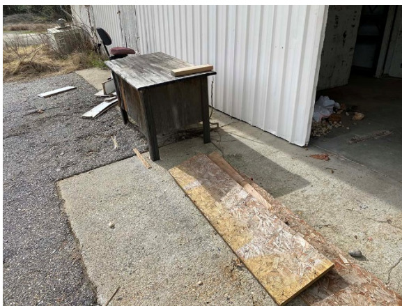
FIGURE 10 - BOARDS WITH NAILS EXPOSED
