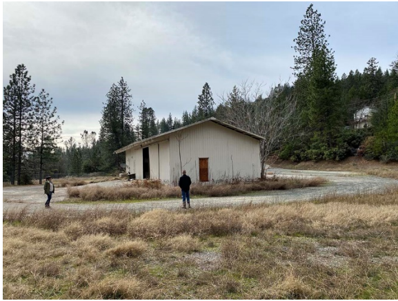
FIGURE 8 - 2ND BUILDING - GARAGE DOOR WIDE OPEN
