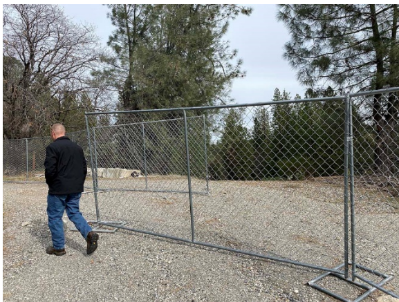
FIGURE 3 - SIDE TOWARDS RR TRACK
