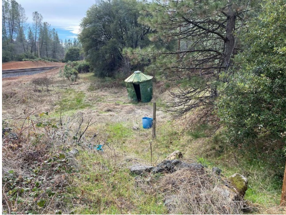
FIGURE 14 - 3RD BUILDING NOT SECURED
