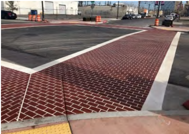
Example Crosswalk Surface Treatment
