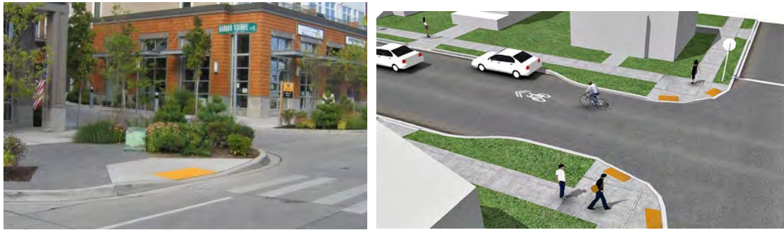
Vegetated curb bulb out (left) and NACTO rendering of a curb extension (right)
