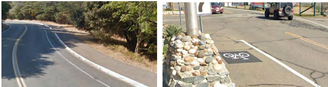
Separated Bikeway (Class IV) along Rising Sun Street (left) and a Class II bicycle lane on Main Street.
