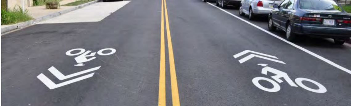
Example of a Class III bicycle route with sharrow markings
