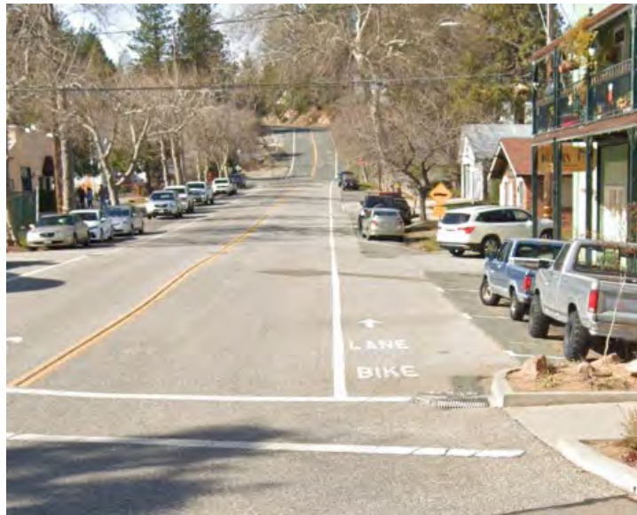
Class III bicycle route on Grass Valley Street (top), Separated bikeway (Class IV) on Rising Sun Street (middle), and Class II bicycle lane on Grass Valley Street (bottom). Source: Google Earth
