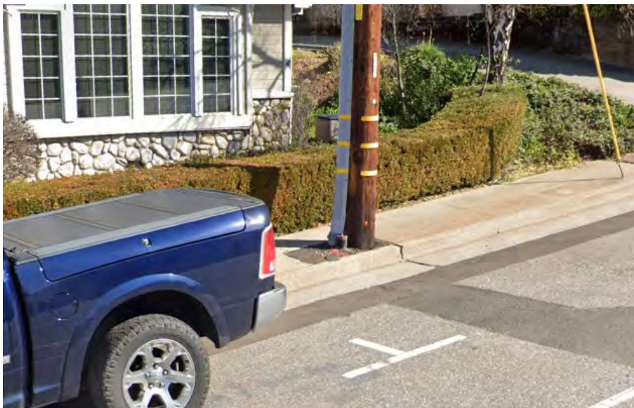
Utility pole on Grass Valley Street obstructing the sidewalk. Source: Google Earth.
