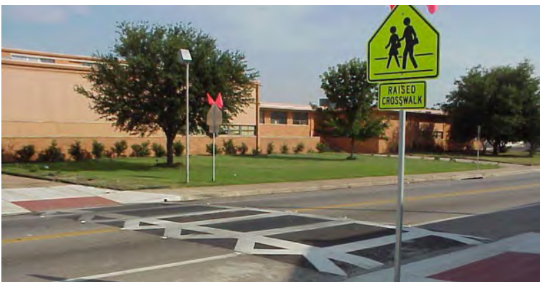
Raised crosswalk at school crossing
