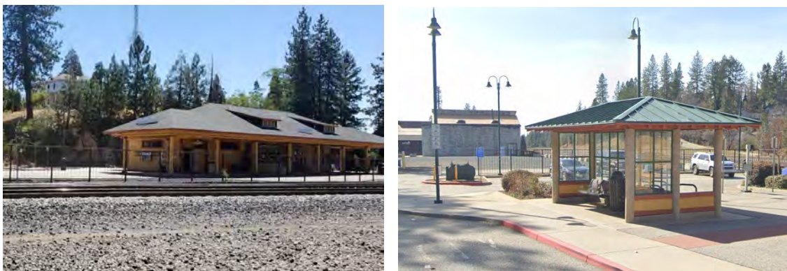
Colfax Amtrak Station (left) and Placer County Transit bus stop (right). Source: Google Earth.
