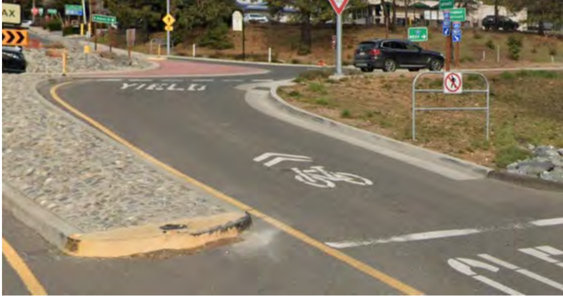
Shared lane markings, or "sharrows," on South Auburn Street approaching the roundabout. Source: Google Earth.
