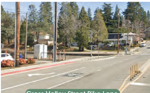
Grass Valley Street Bike Lane
