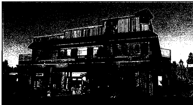
This modern (1972) structure uses historic design elements such as stepped parapet walls, portico with wooden columns, wooden siding with brick panels, and second story balcony.
