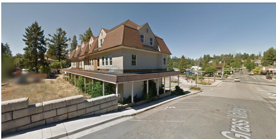
Figure 2: Street view of Northeast building corner
