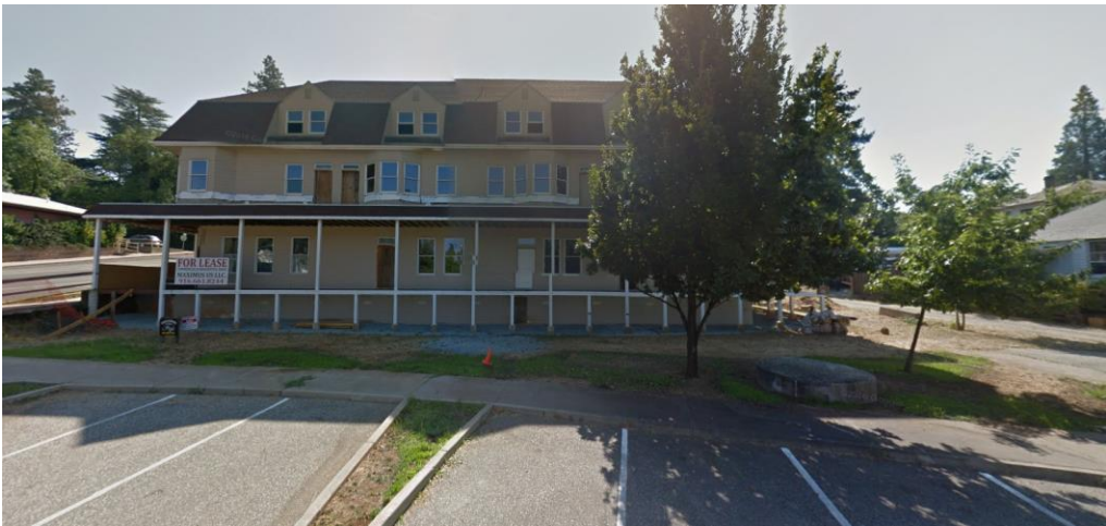
Figure 4: Street view of west side of building
