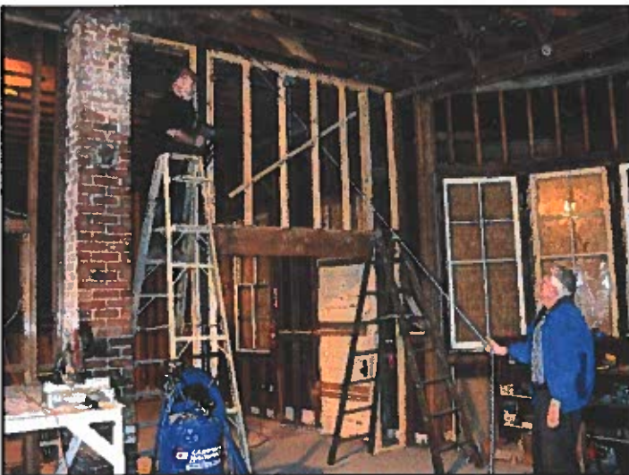
Framing underway for visitor center wall and doorway (left) and waiting room/restroom walls (right)..
