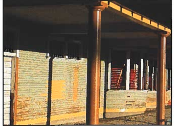
Above - Depot building back on new foundation with repairs where siding was penetrated to move it or removed to bolt it to foundation. Below - Depot building after exterior was prepped and painted.
