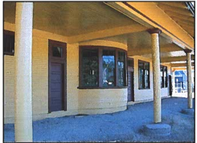
Above - Depot building back on new foundation with repairs where siding was penetrated to move it or removed to bolt it to foundation. Below - Depot building after exterior was prepped and painted.
