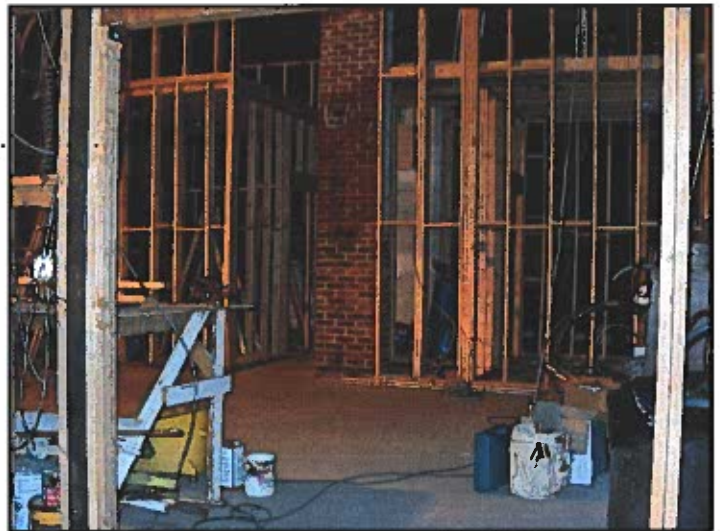
Framing underway for visitor center wall and doorway (left) and waiting room/restroom walls (right)..
