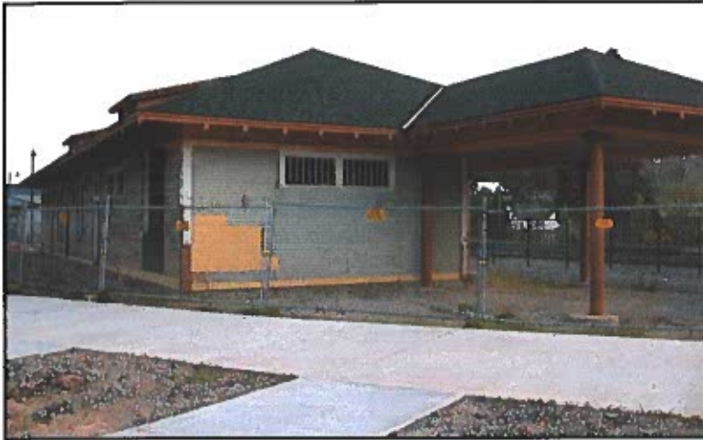
Above - Depot building back on new foundation with repairs where siding was penetrated to move it or removed to bolt it to foundation. Below - Depot building after exterior was prepped and painted.
