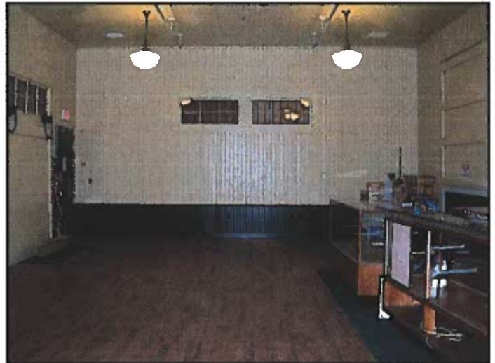
Above left, original boards were reinstalled along with custom-milled replacements. After the room was painted, simulated oak flooring was installed to complete the look. In the photo at right note the operational sliding door at far left next to the new doorway being installed. Simulated wainscot covers new electrical wiring and wall boards that were cut off above the foundation attachments.
