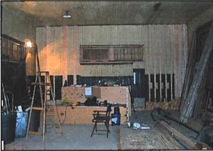
Above left, original boards were reinstalled along with custom-milled replacements. After the room was painted, simulated oak flooring was installed to complete the look. In the photo at right note the operational sliding door at far left next to the new doorway being installed. Simulated wainscot covers new electrical wiring and wall boards that were cut off above the foundation attachments.
