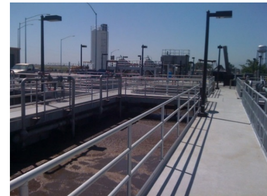
DVI WWTP Tracy
