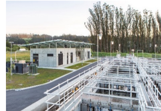
USCG Tracen WWTP
