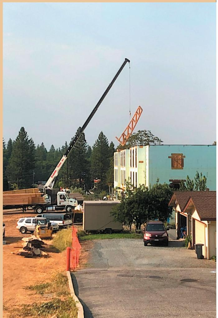
**Roof trusses being hoisted up on the Best Western Motel project. Photo by Alan Shuttleworth**
