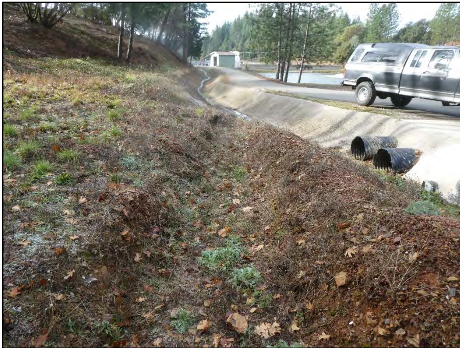
The ephemeral stream drains into a concrete lined channel along the eastern boundary of the WWTP area.
