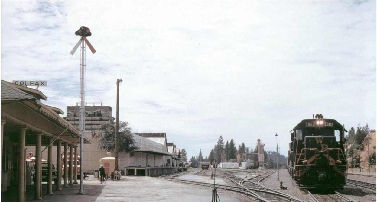
The semaphore type signal in front of the Colfax Depot in the diesel era
