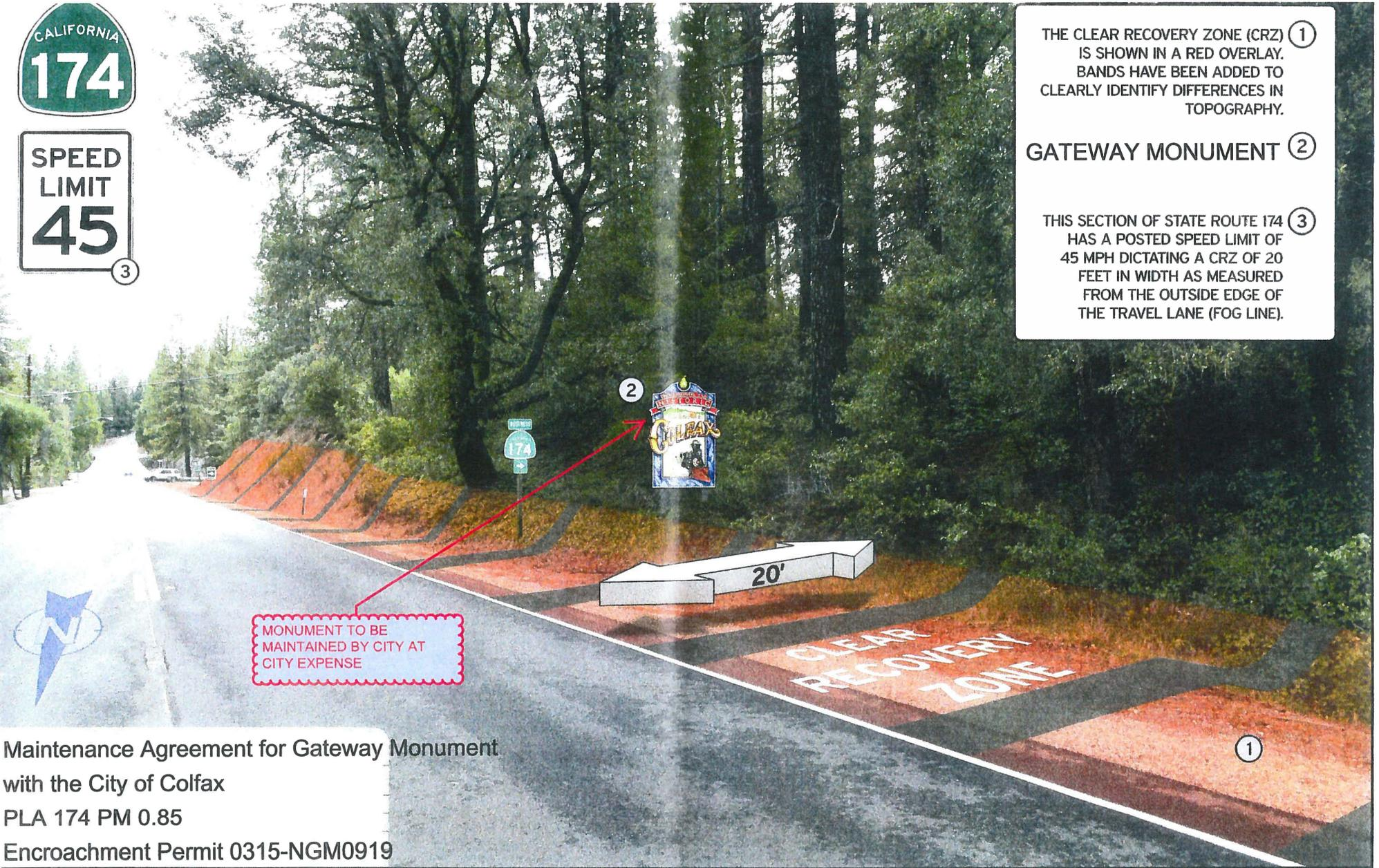
THE CLEAR RECOVERY ZONE (CRZ) ① IS SHOWN IN A RED OVERLAY. BANDS HAVE BEEN ADDED TO CLEARLY IDENTIFY DIFFERENCES IN TOPOGRAPHY.
