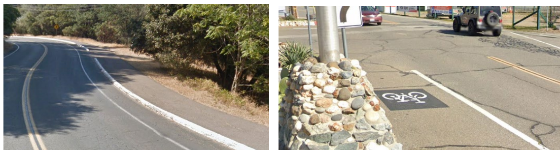
Separated Bikeway (Class IV) along Rising Sun Street (left) and a Class II bicycle lane on Main Street.
