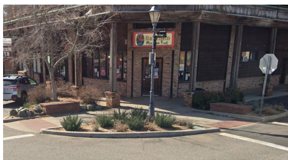
Curb ramps with curb extensions on Main Street and Grass Valley Street (left) and bypass ramp on Main Street. Source: Google Earth.
