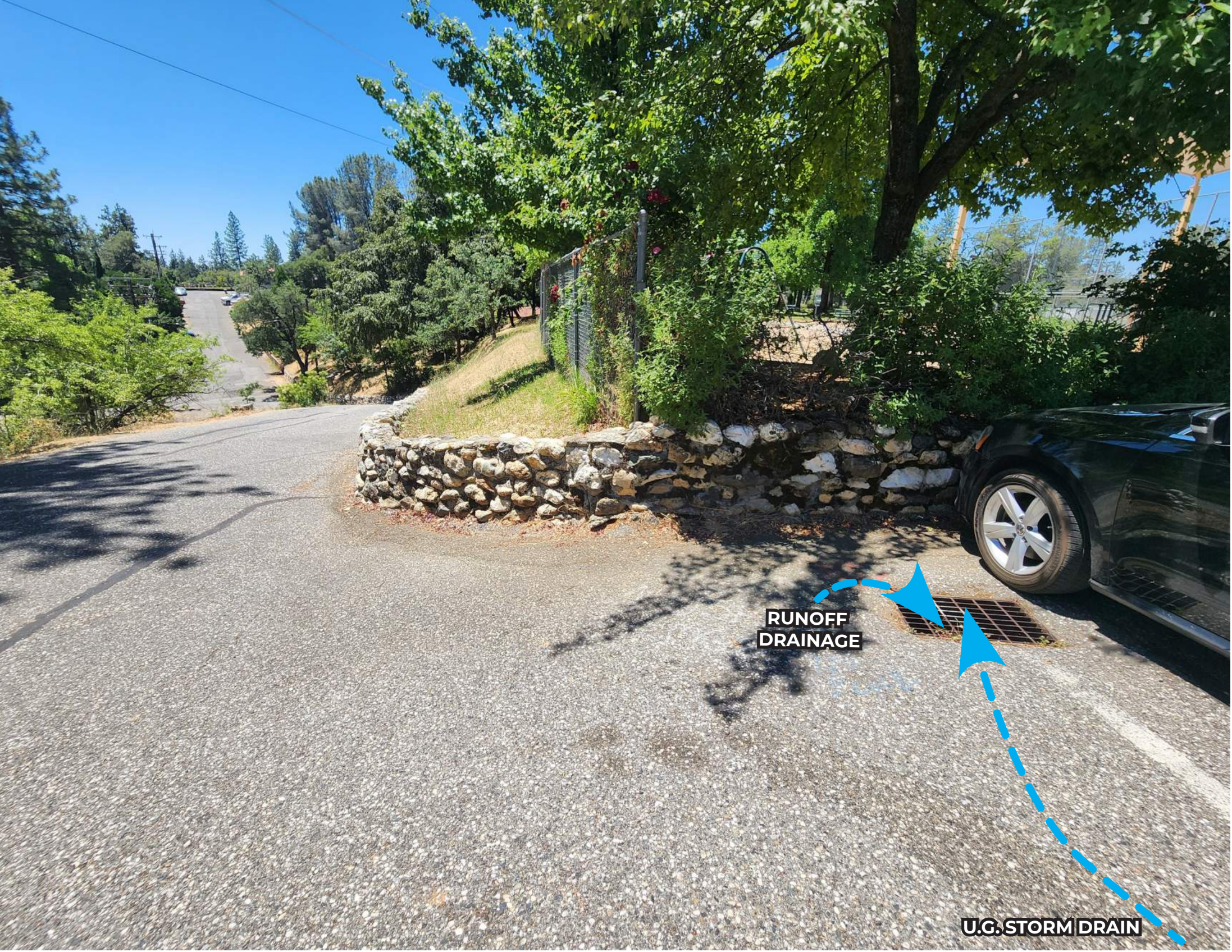
STORM DRAIN WATER LINE POINT OF CONNECTION
