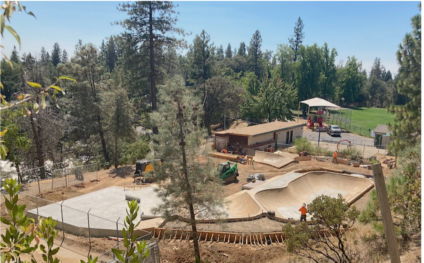
After 15+ years of public discussion, a skate park begins taking shape where Colfax once had a community swimming pool. October 3 will be opening day for the park. Photo by Will Stockwin
